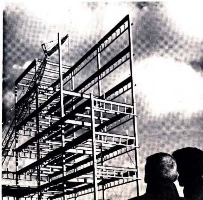
AIR CONDITIONED—RIT students marveled at the new style air conditioning that will add a mark of distinction to the new Nathaniel Gleason Hall.
