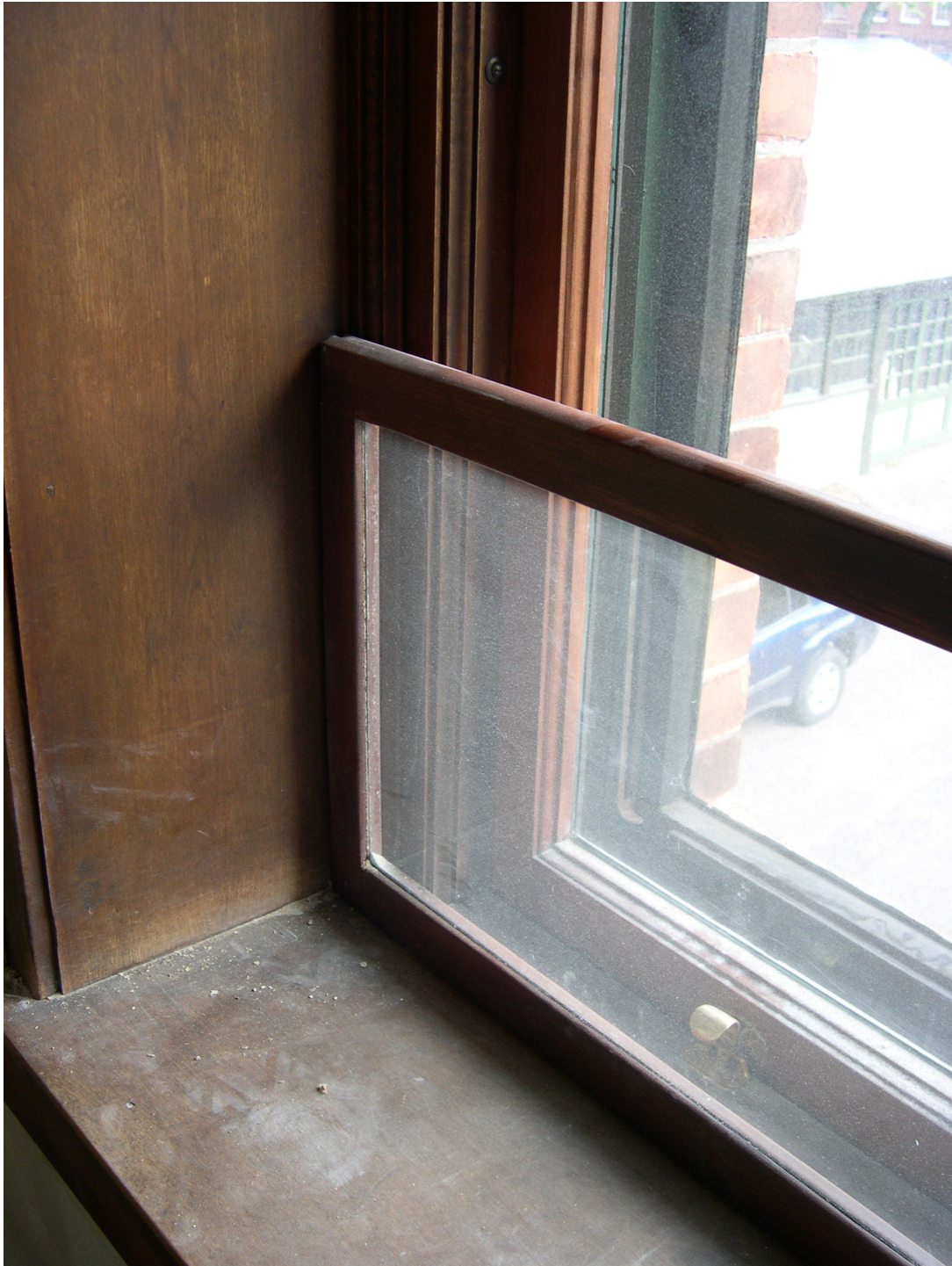
Figure 3.14: Window in the C&H Drafting Room, with extra window pane to prevent wind-scattered papers. In situ, Calumet and Hecla Mining Company Office Building, Calumet MI. Photo by Eric Nystrom, 2006
