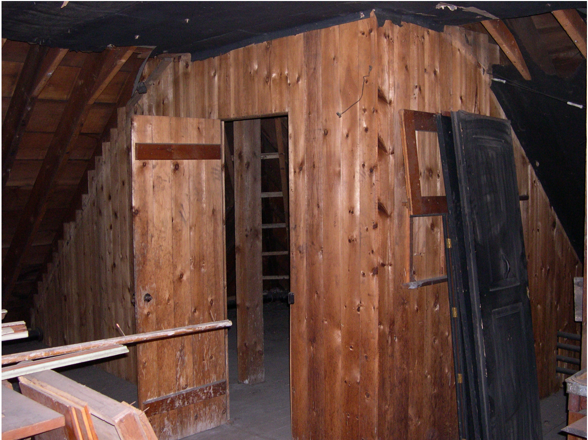
Figure 5.4: The Quincy Mining Company constructed a darkroom by walling off a portion of their office building's attic. In situ in the Quincy Mining Company office building, Keweenaw National Historical Park, Hancock, MI. Photo by Eric Nystrom, 2006.
