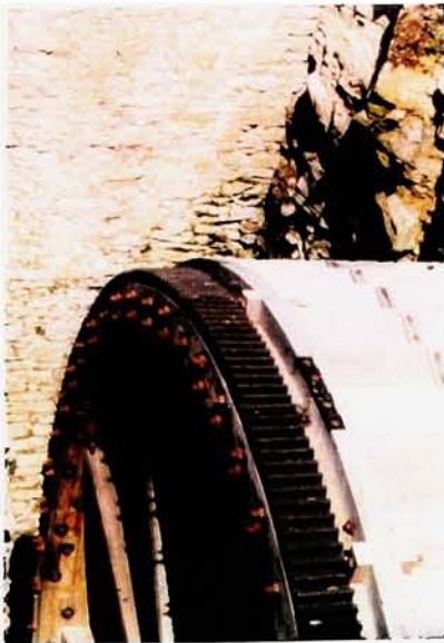
the water wheel c. 1840
