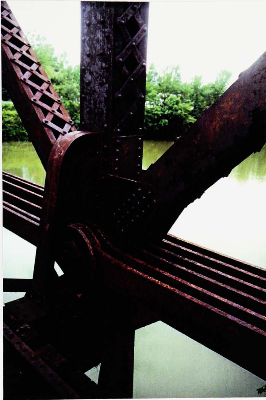
Train Trestle Detail (Henrietta, New York)
