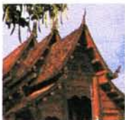
Triangle gable and multi-tiered roof
