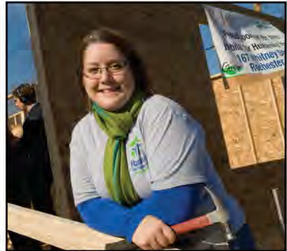
Kaity Werner on site at RIT's sustainable home project. (Photo by A. Sue Weisler '93)
