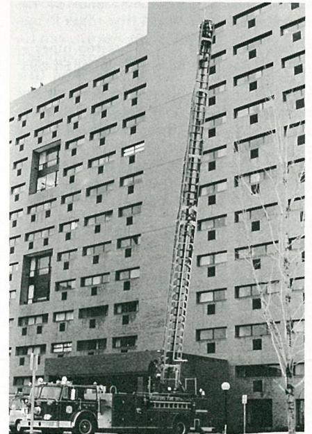
A 100 foot ariel hook-and-ladder fire truck from the Pittsford fire department was used in a fire drill last Sunday afternoon at the 12 story NTID dormitory. It was the first fire drill at the high tower using actual equipment.
