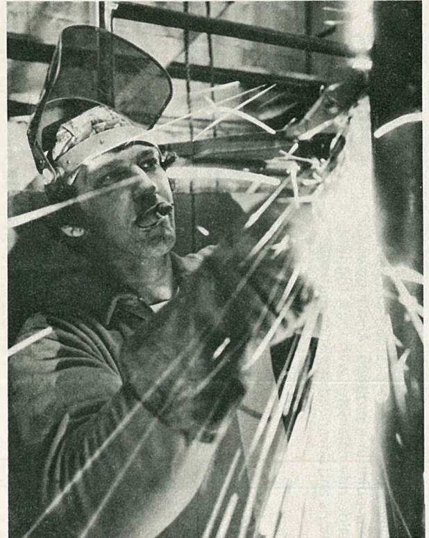
A workman smooths welds on the main stairway railing.
