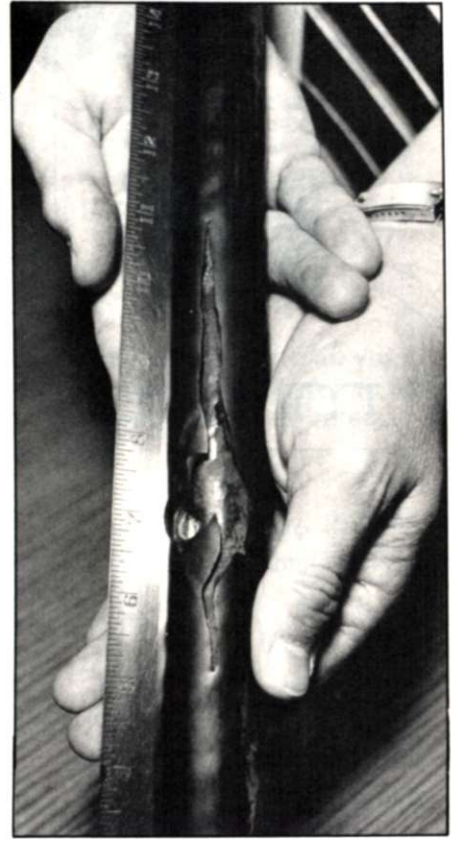
The culprit (right). The original cracked piece of cable which halted classes in three academic buildings.
