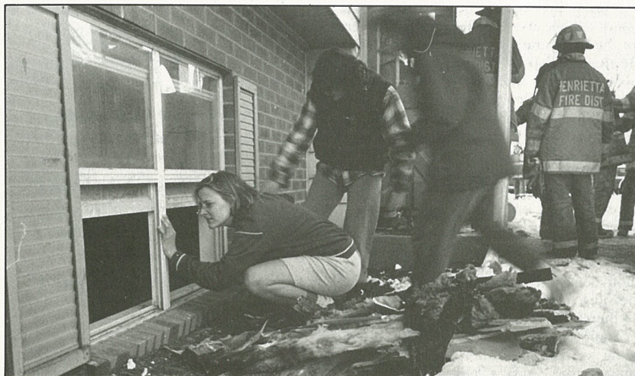
Residents of 277 Perkins inspect the damages incurred after a fire broke out the afternoon of March 28.
