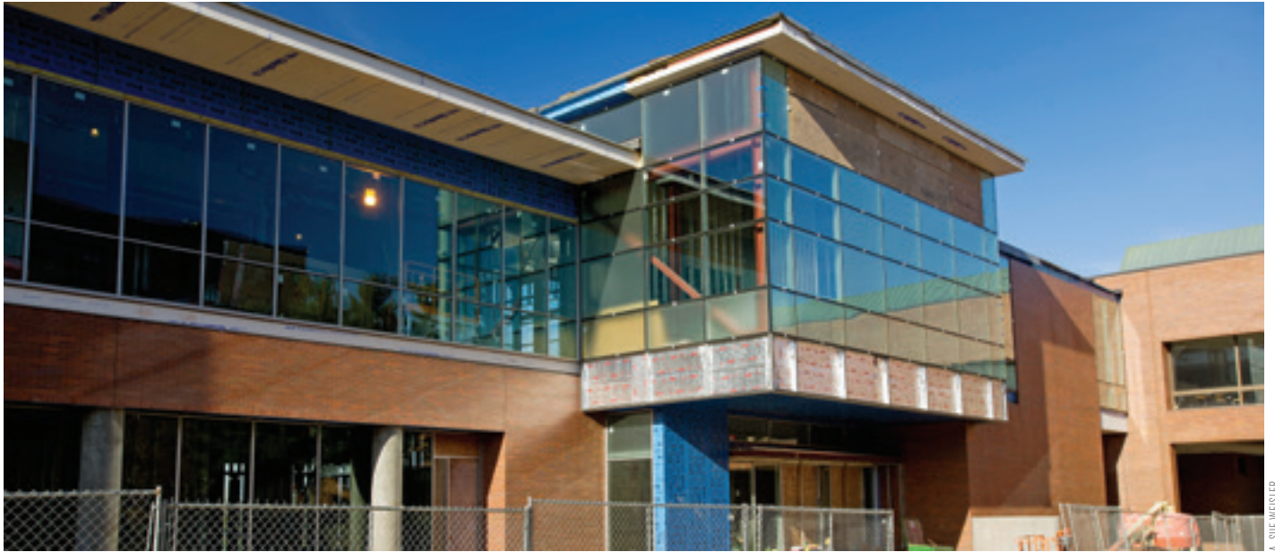
Creating an Innovative Space Construction continues on Sebastian and Lenore Rosica Hall, slated to open in October.
