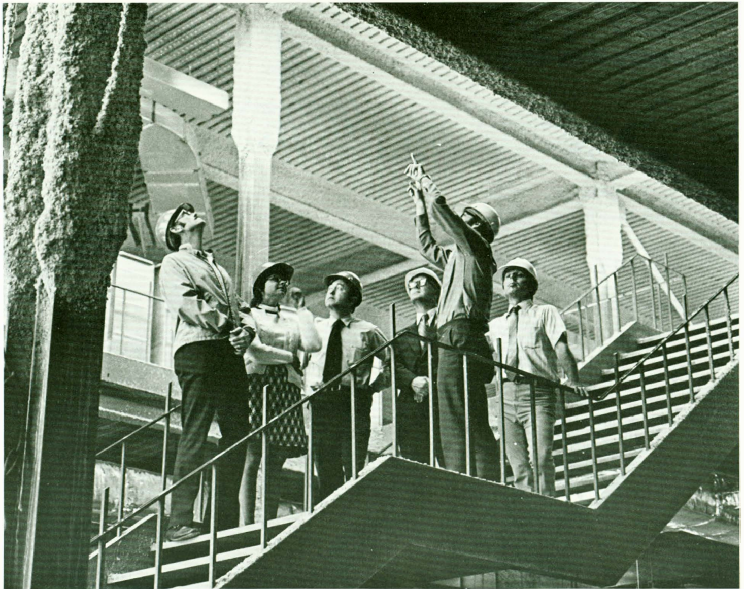
CLOSE INSPECTION —William Williams, assistant to the director of NTID, explains special construction features, such as fireproofing for steel girders, to staff members (from left) Joe Avery, Jane Bolduc, Jim Collins, John Kubis, Williams and Lou Boyon, construction supervisor.
