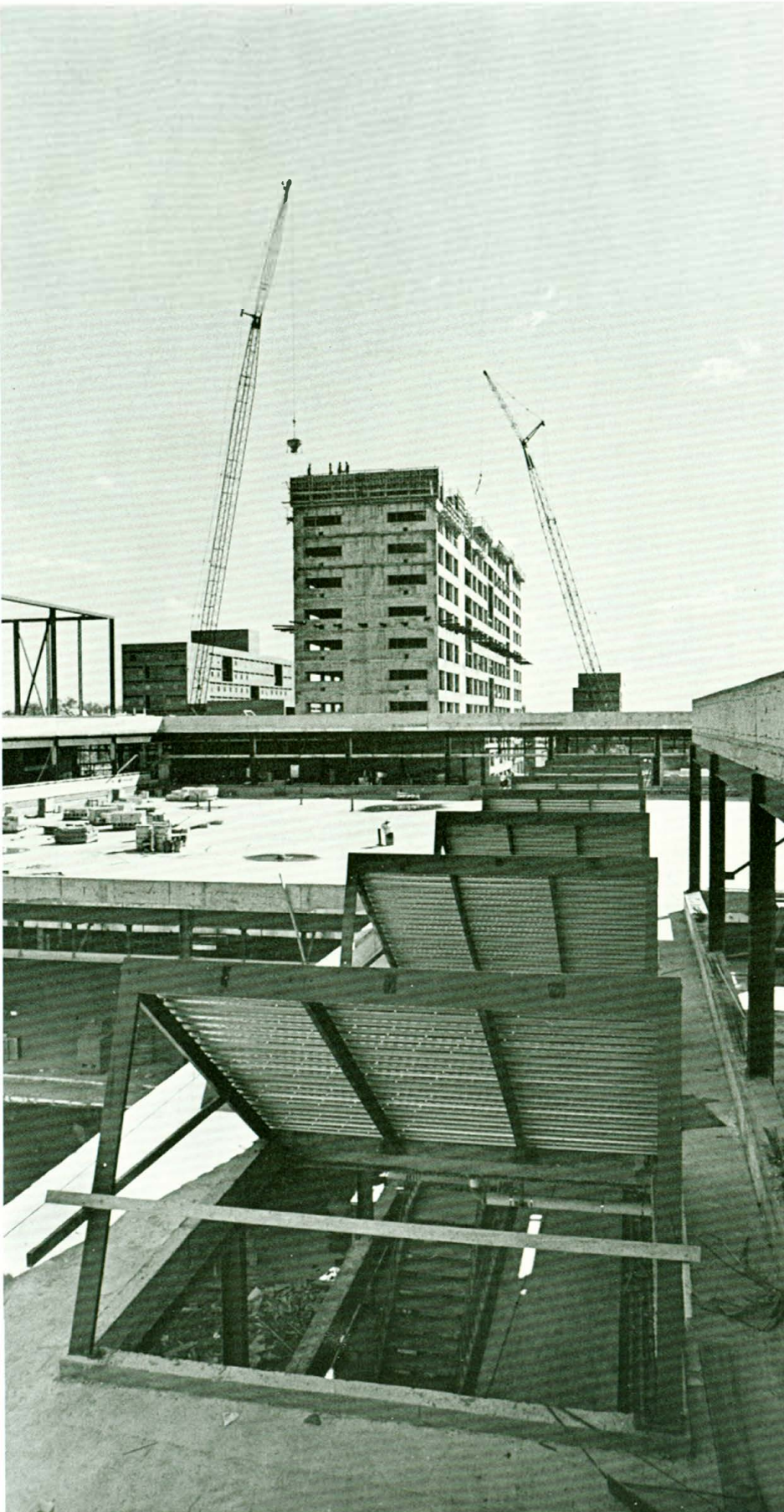
TO LIGHT STREET —Skylights in the academic building will light the "internal" street with northern non-glare light.
