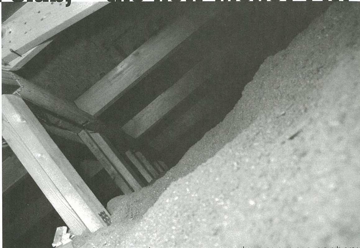
Racquet Club attic space--insulation, sawdust, or the Sahara?
