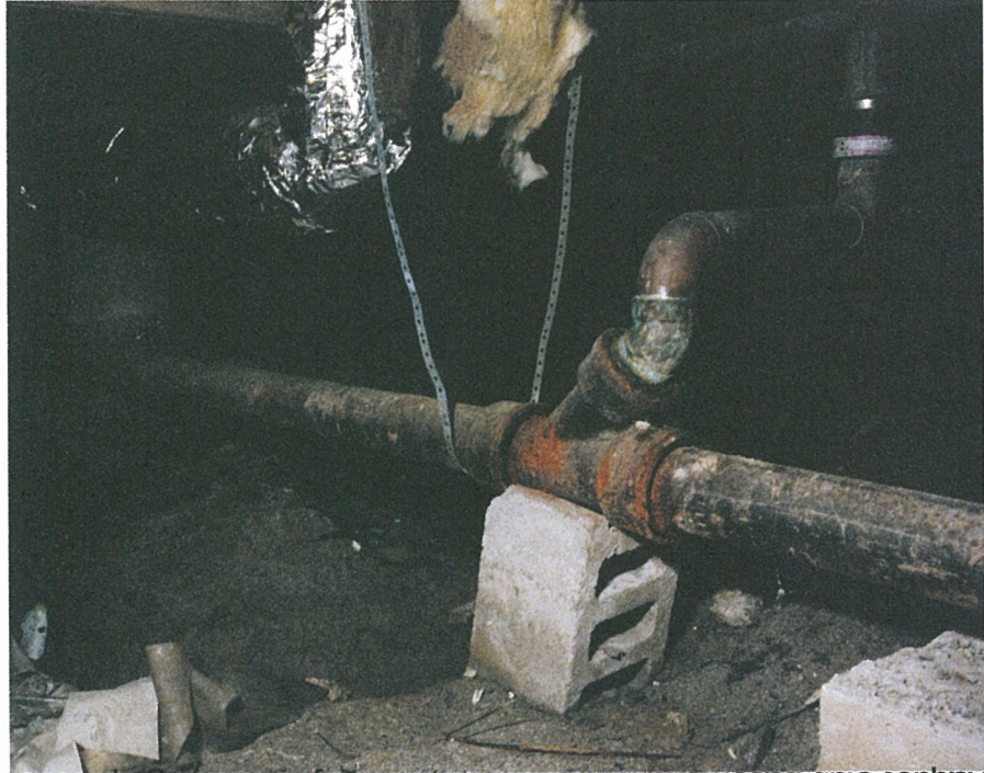
Racquet Club basement--cinder blocks, not only for holding up beds.
