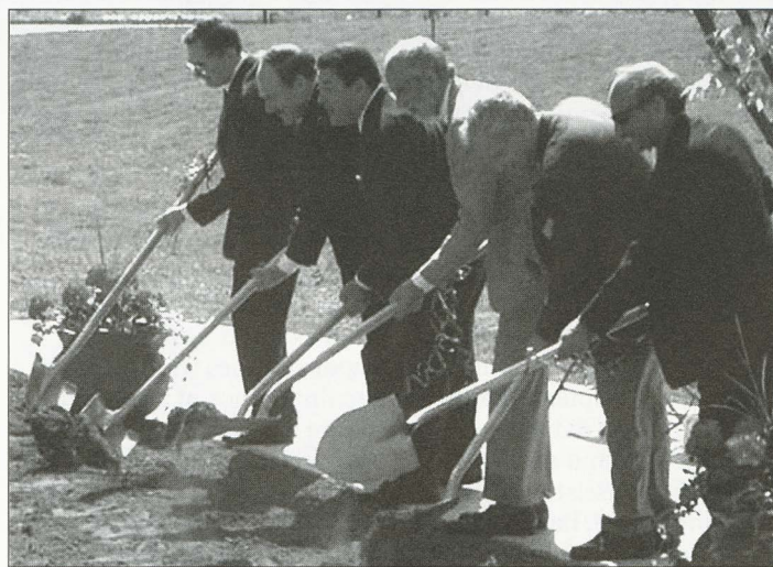
CEREMONIAL GROUND BREAKING... At a groundbreaking May 10, RIT President Simone; Frontier CEO Martin Mucci; Sen. Jim Alesi; Don Boyd, IT Collaboratory director; Walter Wolf, acting dean; B. Thomas Golisano College of Computing and Information Sciences; and Jeffrey Lasky, head of the IT Lab, break ground for the new cutting-edge facility designed for research and development. Alesi was instrumental in securing the $1.5 million funding for the IT Lab.
