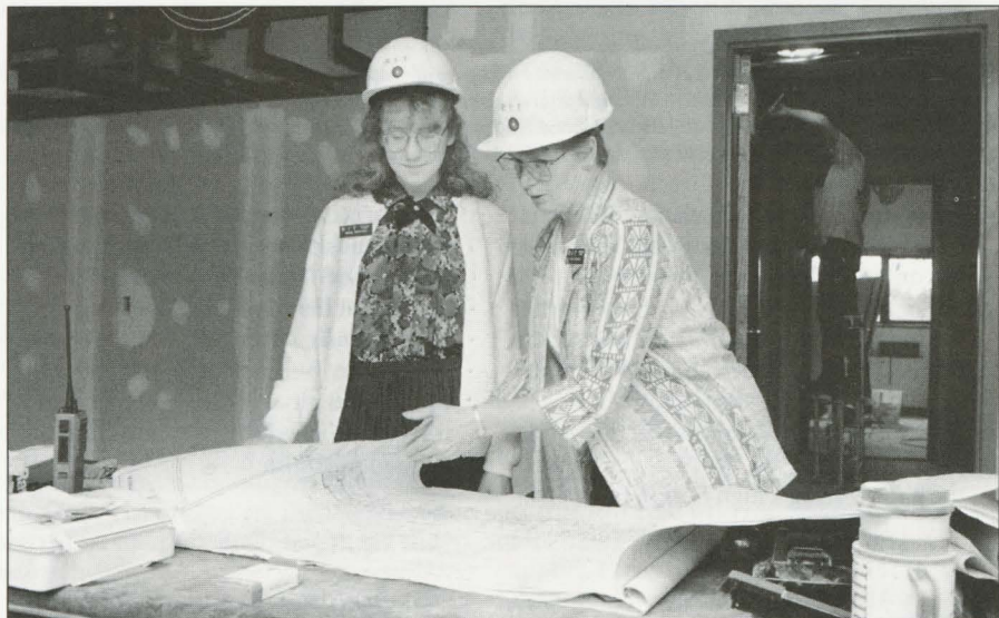
HELPING GIRLS SEE THEIR FUTURE... Carol Schmitz, construction/projects manager for Physical Plant, shows Halina Shkavritko, a Jefferson Middle School student, the plans for Margaret's House, RIT's new child care center in Alexander Graham Bell Hall. Take Our Daughters to Work Day, April 25, was filled with experiences like this one for young girls.
