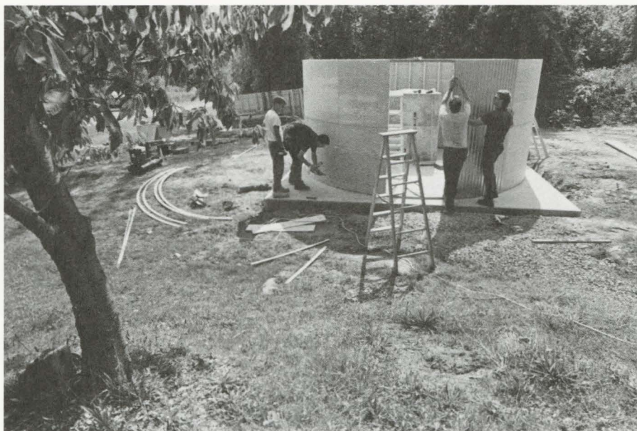
AREN'T THERE ANY CORNERS? . . . Thanks to the efforts of Physical Plant workers, RIT has a new astronomical observatory. The round building has a five-meter dome roof and will house a reflecting telescope with a 16-inch-diameter mirror, expected to arrive this month. The observatory is mostly funded by the National Science Foundation and is a shared project between the College of Science and the Center for Imaging Science. Viewing should begin in Winter Quarter.
