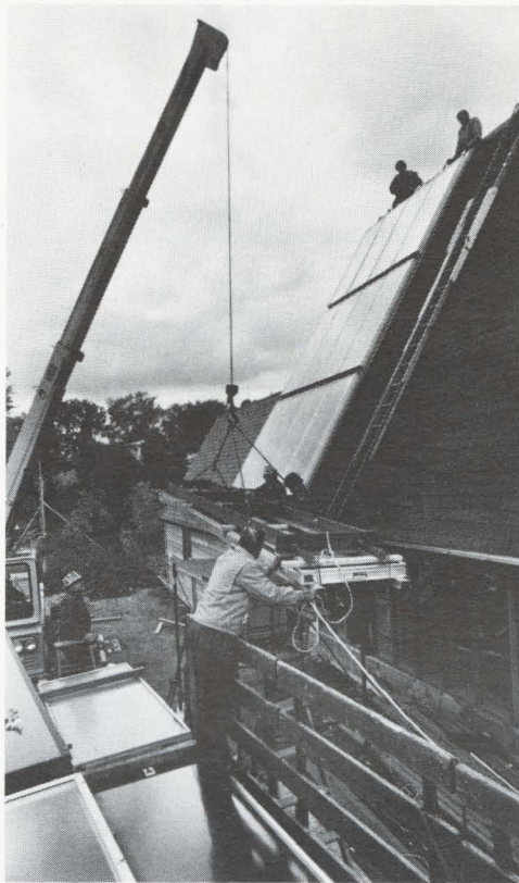
THE PANELS GO UP!
