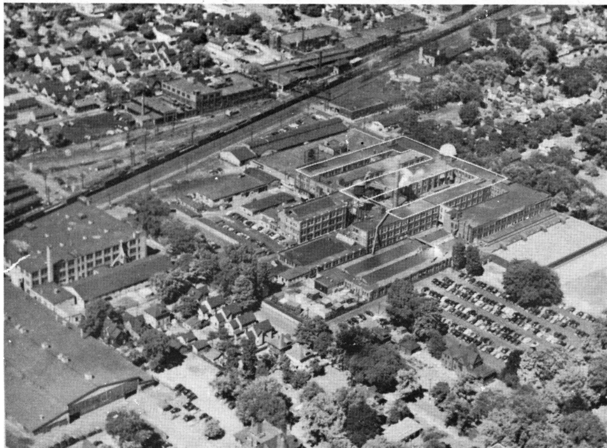
The present Taylor Instrument Companies' plant in Rochester is shown above. The white line represents the area of the original plant built in 1905. Instruments in themselves are not very large, yet it takes 400,000 square feet of floor space in which to perform all of the many steps necessary to produce the finished product.
