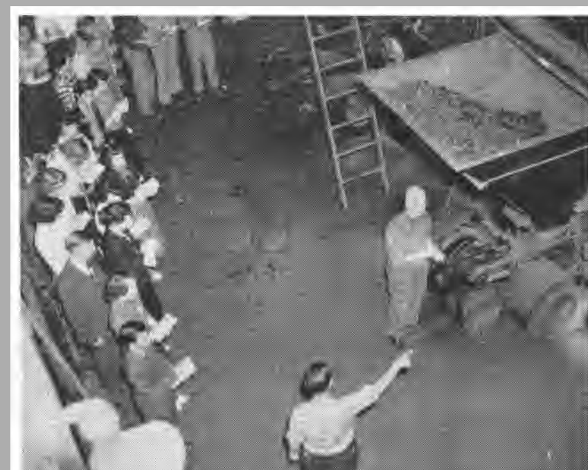
General Science classes visit the school's boiler room for practical observation of its operation, a tie-in with the thermal technics studies. Visual insight into the practical application of subjects covered in the classrooms has proven beneficial to the students.
