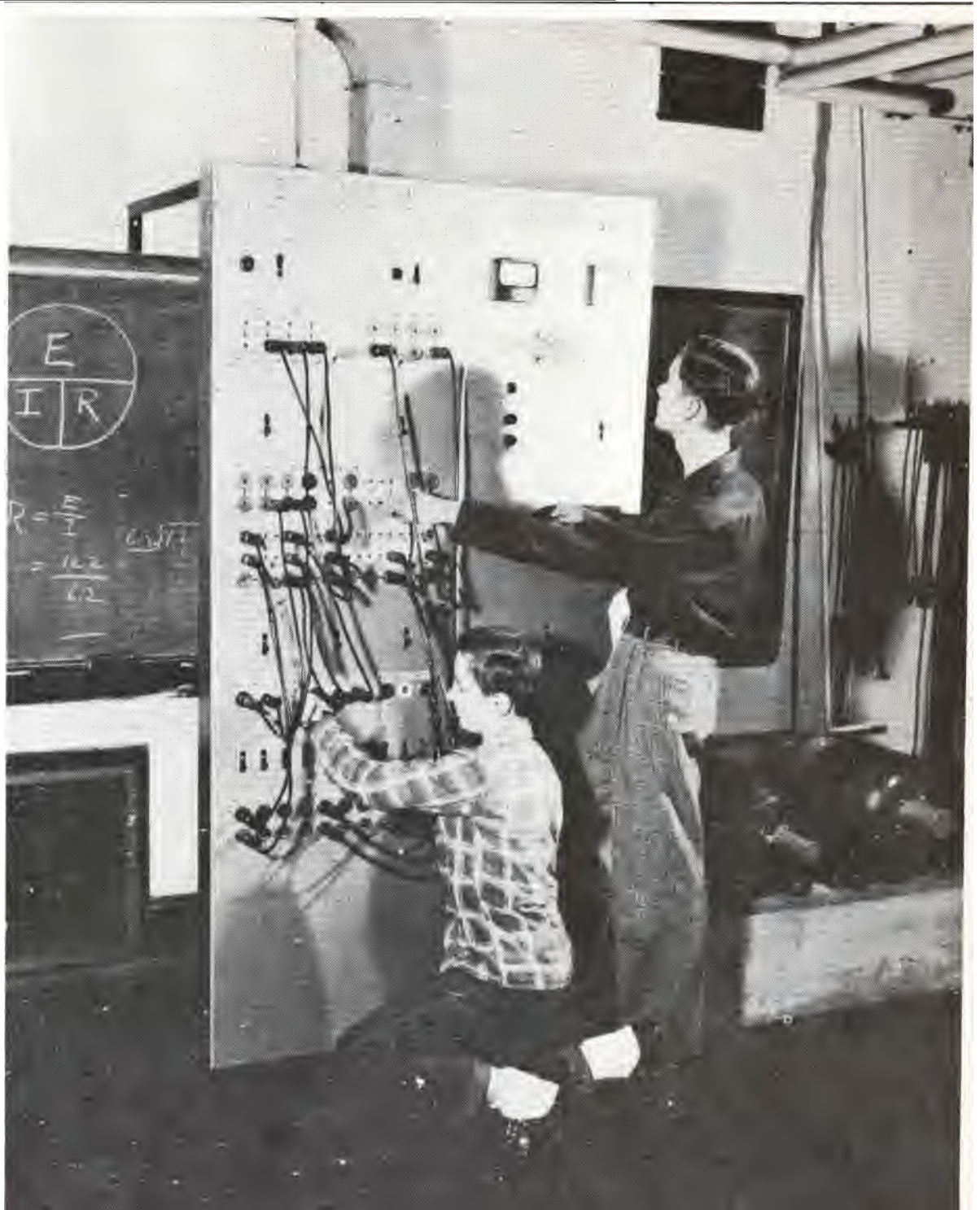
Jerry Schatiner and Anthony Scott work in the electrical lab on a new control and distribution board. Edison's electrical department is one of the most elaborate.
