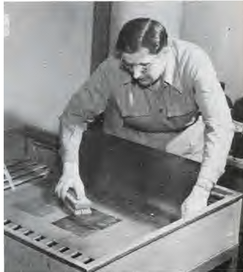
Offset procedures are explained and carried on by students in the offset laboratories. Here a student is shown preparing a zinc plate for production in the offset pressroom.
