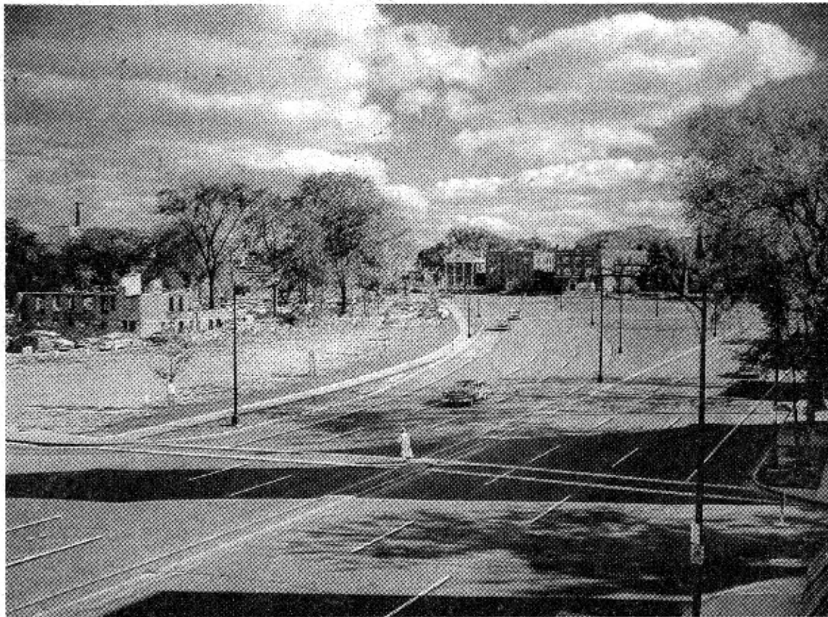
DOWN PLYMOUTH AVENUE—Located near the center of Rochester, RIT is within walking distance of downtown stores, theaters and other points of interest. Eastman Kodak and other industries add to
