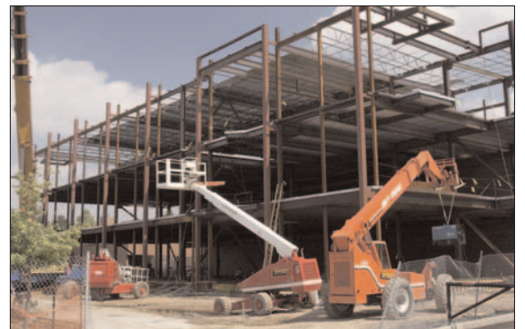
Springtime saw the IT Collaboratory building begin to take shape.
