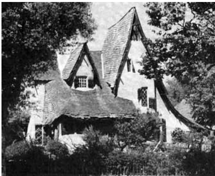
House used on various film sets The Spadena House, Beverly Hills, CA
