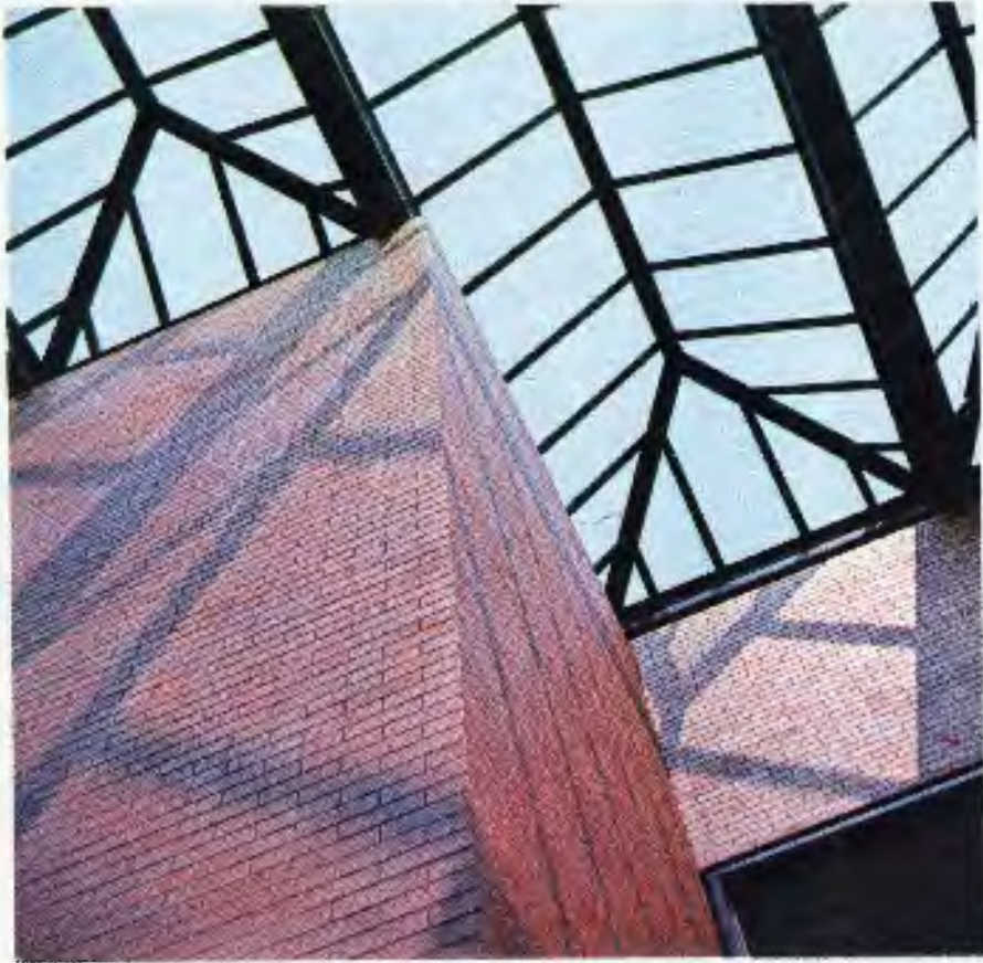
Looking up at glass windows between the gym and ice rink.
