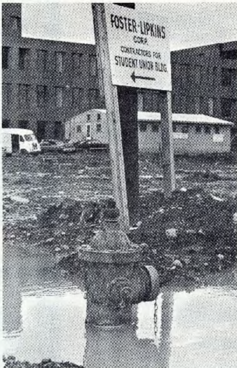
BOGGED DOWN —A direction sign of Foster-Lipkins, contractor of the behind schedule College Union and Graphic Arts buildings at the new campus, seems to typify that firm's completion lag. (Staff photo by Nick Morgan)
