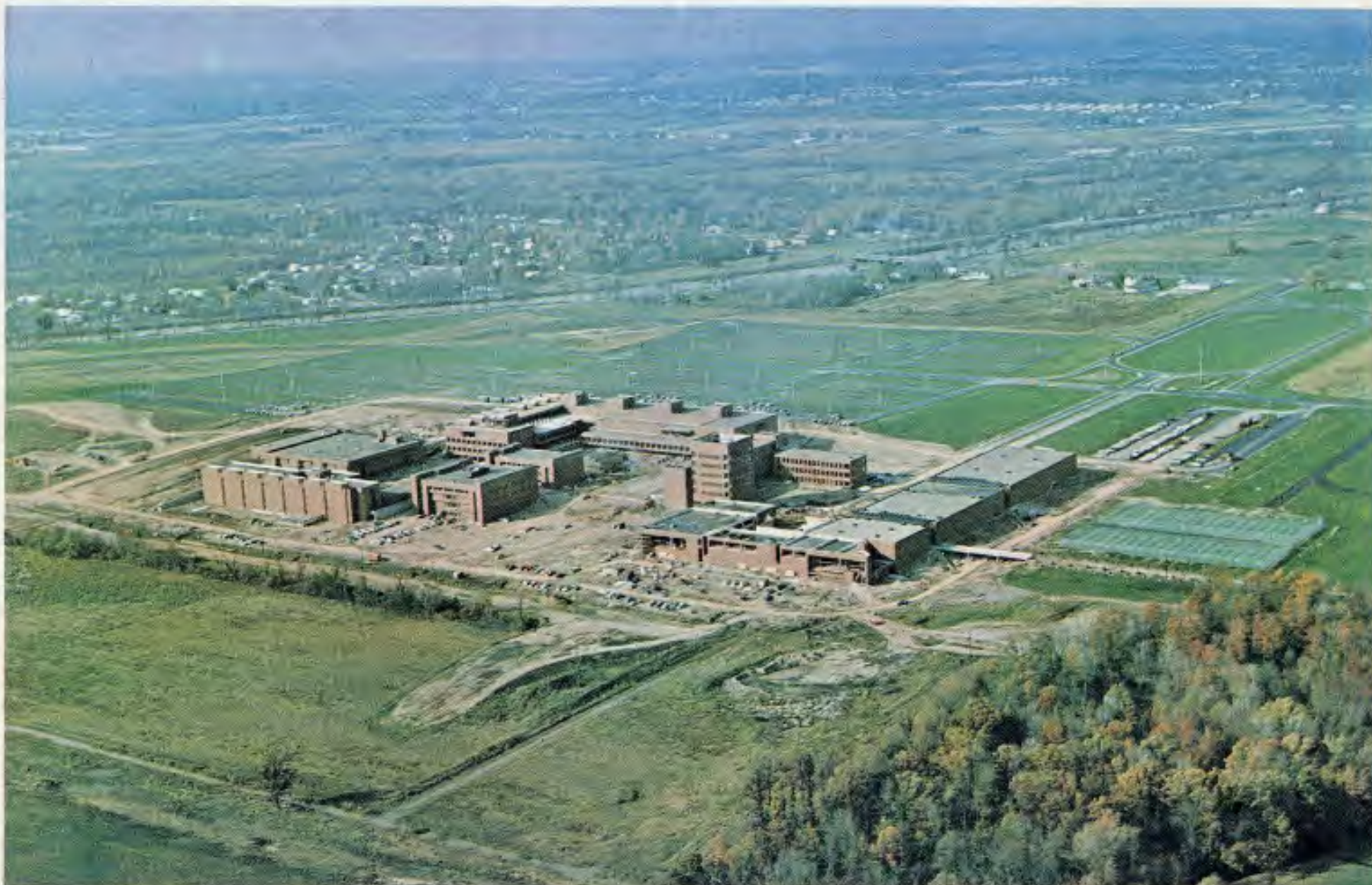
ACADEMIC COMPLEX —This over all view of the new RIT Campus illustrates the final stages of exterior construction. The College Union building (lower right corner of the complex) and the Graphic Arts and Photography Building (center rear) are the least completed structures. The now occupied Administration Tower, located in the center of the complex, has undergone interior painting and decorating. The Physical Education Building (far right), housing the swimming pool, ice rink and gyms, is almost ready for interior decorating. The most complete of all the new campus structures is the Applied Science Building (lower left). As of this issue, all that remains before occupancy of this building is possibly the installation of chemicals, equipment.
