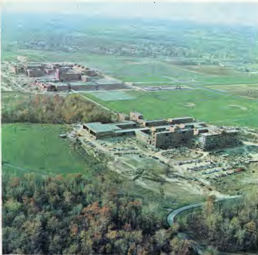
STUDENT HOUSING —The housing complex in relation to the academic buildings is shown above. Dividing the two areas is a pathway about as long as a football field. No, classes won't be called because of rain or snow.
