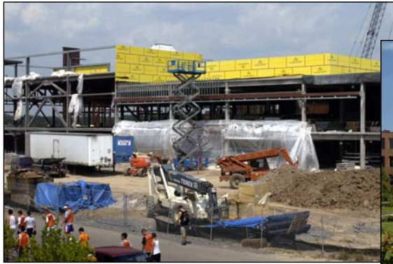
RIT's newest addition, The Field House and Activities Center
