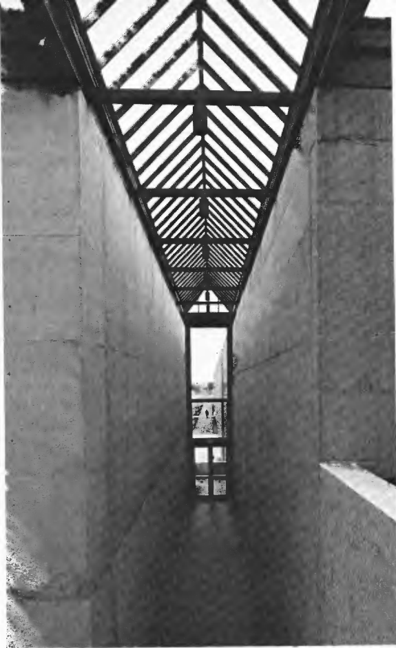
view of the side exit in the College Union building
